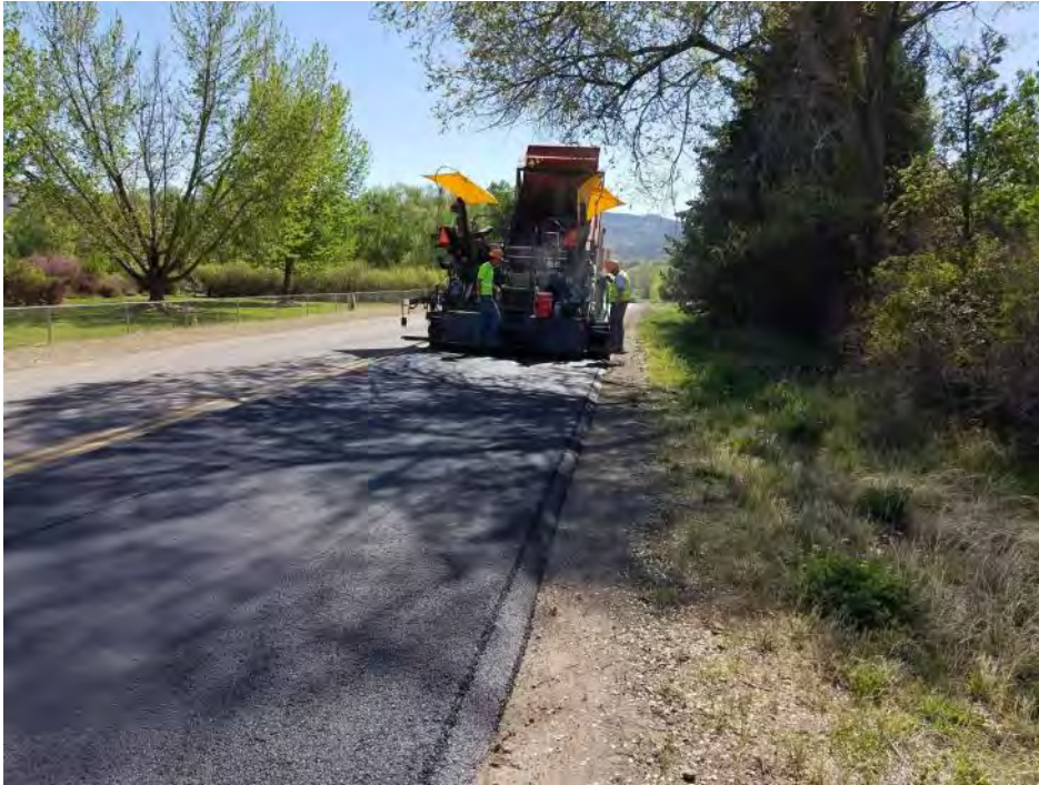
Courtesy photos above and right of county crews performing asphalt overlay operations with the safety edge on Uncompaghre Road.
